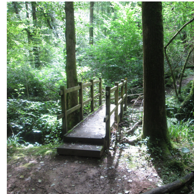
5. The wooden bridge
