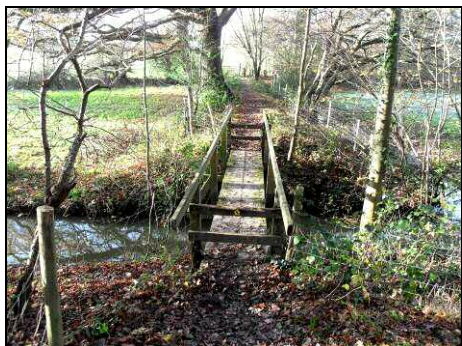
Pic 3: The wooden footbridge
