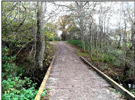
Pic 3: The wooden bridge
